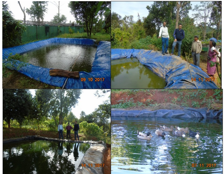
Jalkund a low cost water harvesting structure
